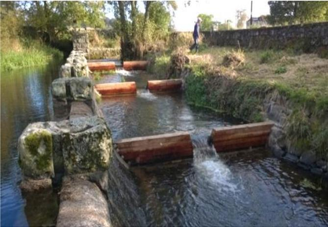
Loch of Skene – pool and weir fish pass
